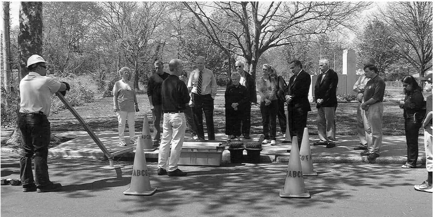
Assemblyman Bob Sweeney is pictured here with officials from the Village of Lindenhurst, and members of the Sierra Club and SPLASH (Stop Polluting, Littering and Save Harbors), reviewing the installation of a new storm basin filtering system to prevent pollutants from flowing into local ponds. This system will help filter storm water runoff and reduce the harmful pollutants in the water.
